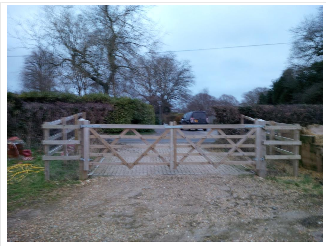
View of new access gates.
